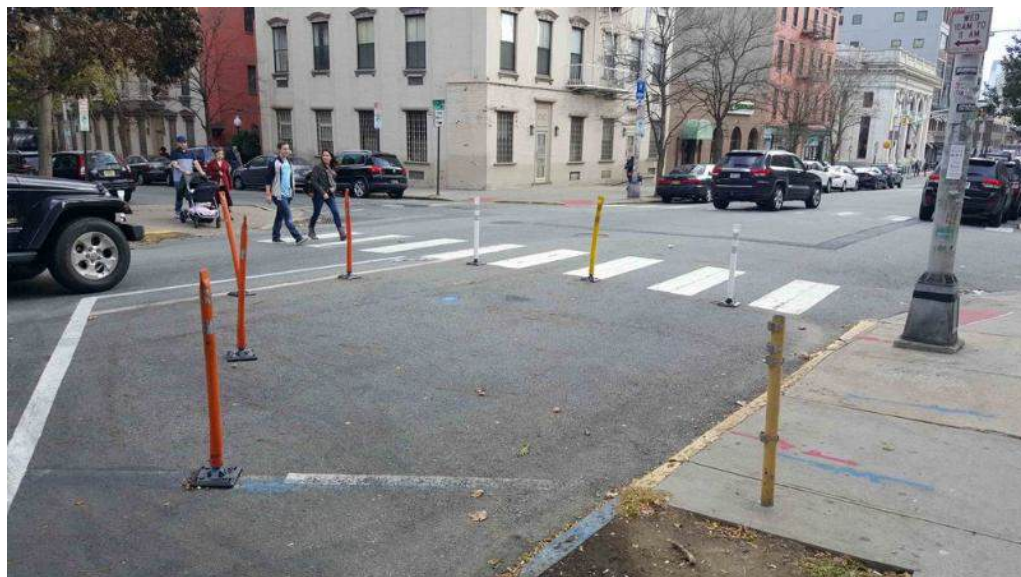
Figure 40: A low-cost bump-out has been created using flexi-post bollards (Source: Strong Towns)
